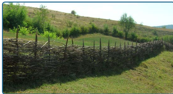
Figure 4. Example of fencing in the field (Photo: Ivalsa)
