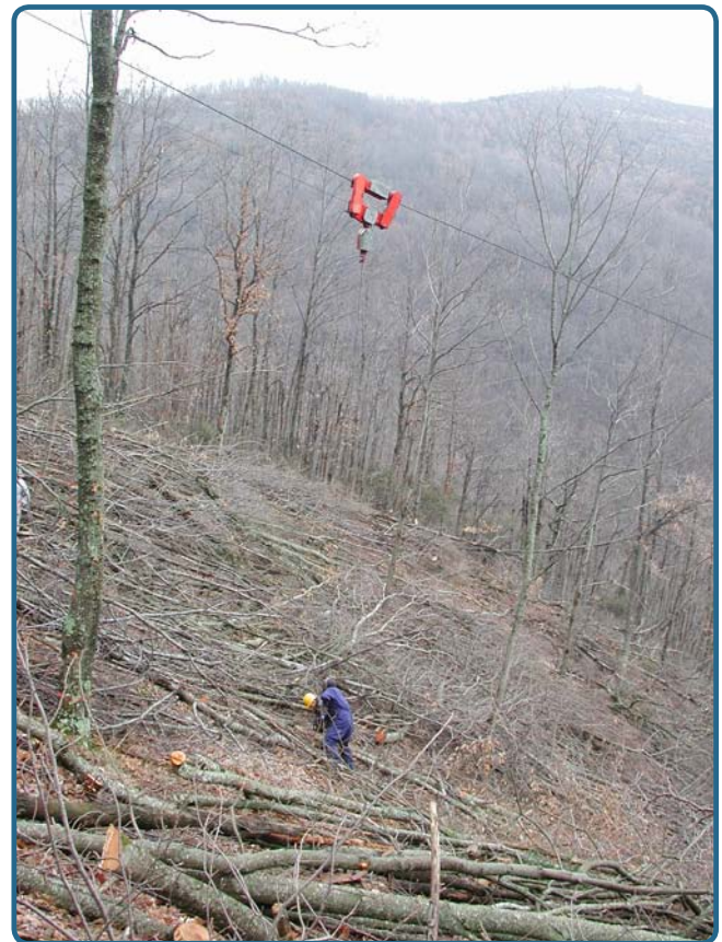
Figure 6. Cable yarder extraction is the best solution when site conditions are not favourable to machine access (Photo: R. Spinelli)
